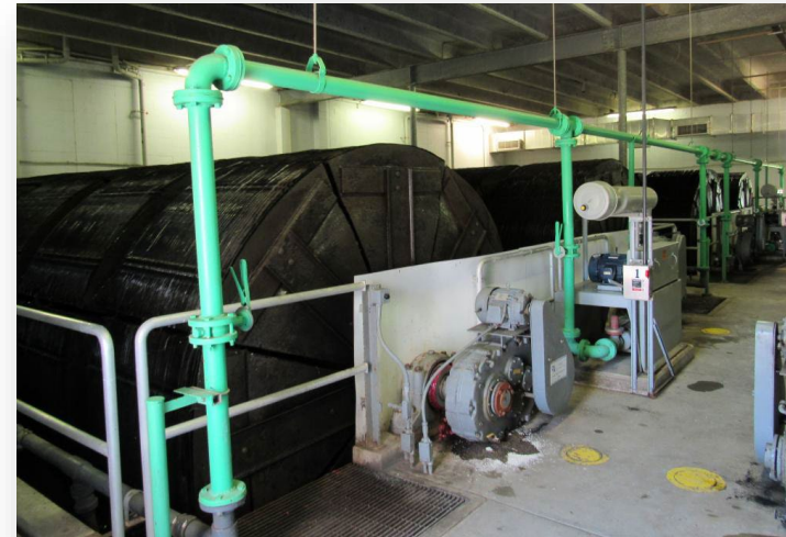
Figure 7. Rotating Biological Contactor (RBC)
